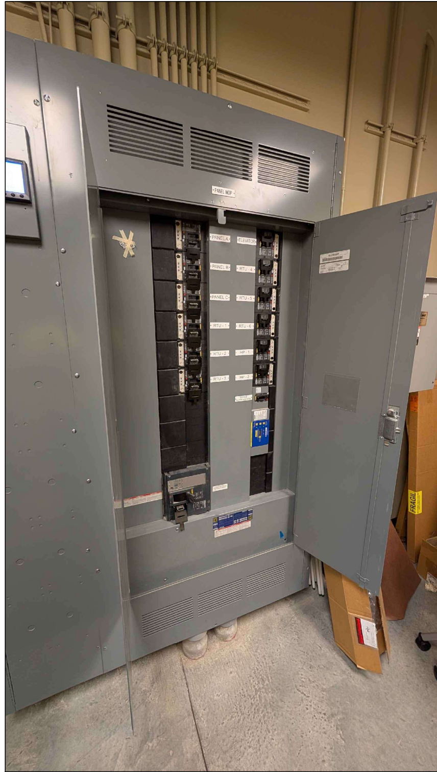
2 EXISTING MDP BREAKER LAYOUT (RM 119 - LOOKING EAST) E2.1 NTS
