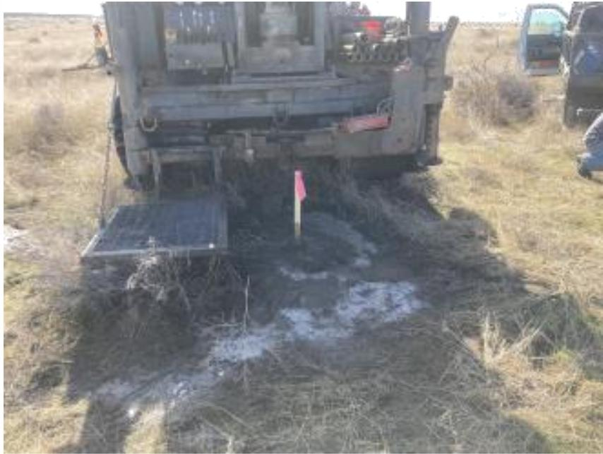
**Photo 2** - Example of bentonite-backfilled borehole
