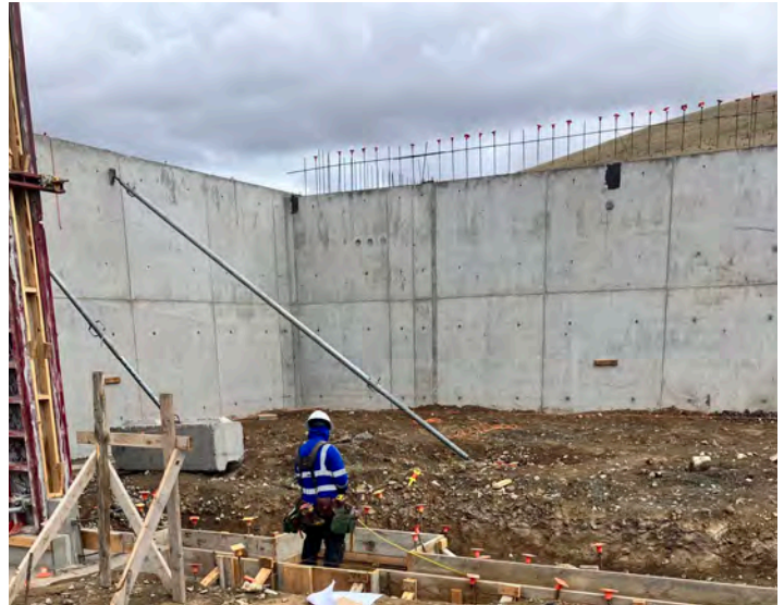
SilverCreek's concrete crew forming the south continuous footing on level 1.
